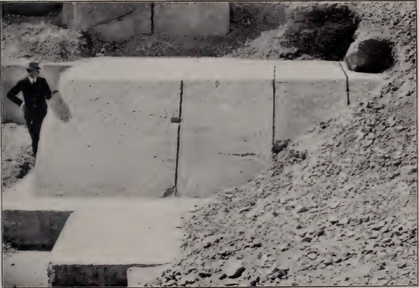
FIG. 66.—CASING BLOCKS AT THE BASE OF THE GREAT PYRAMID. JOINTS OTHERWISE UNDISCERNIBLE INDICATED BY CHARCOAL LINES. (Photograph by L. D. Covington.)
